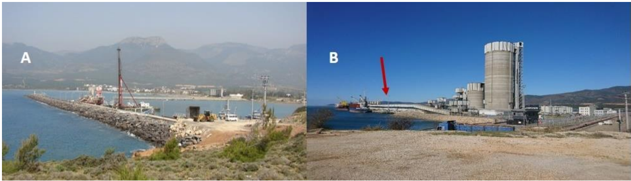
Figure 12. The port before (A) and after (B) construction (arrow shows new pier).
